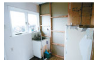
Laundry showing end wall to kitchen before removal.
