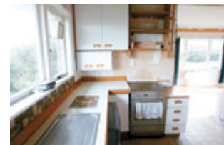
Kitchen showing end wall to lounge before removal.
