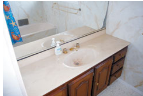
Before (right and below pics) of the bathroom.
