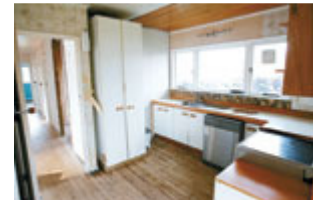
Kitchen showing end wall to laundry before removal.
