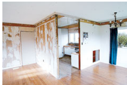
Lounge/kitchen before removal of wall on right.
