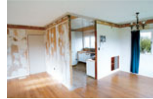
Lounge/kitchen before removal of wall on right.
